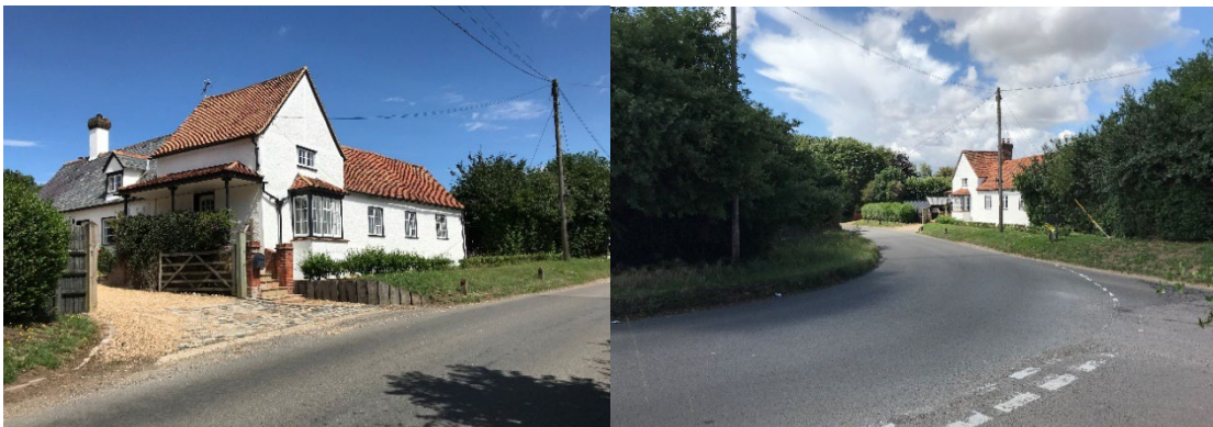
Chequers and view towards the property from the south-west boundary of SW2
