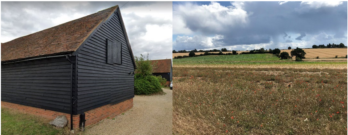
Old Farm Buildings/Barn and Hovel at Bancroft Farm. View towards the roofs of the buildings from the Main Site.
